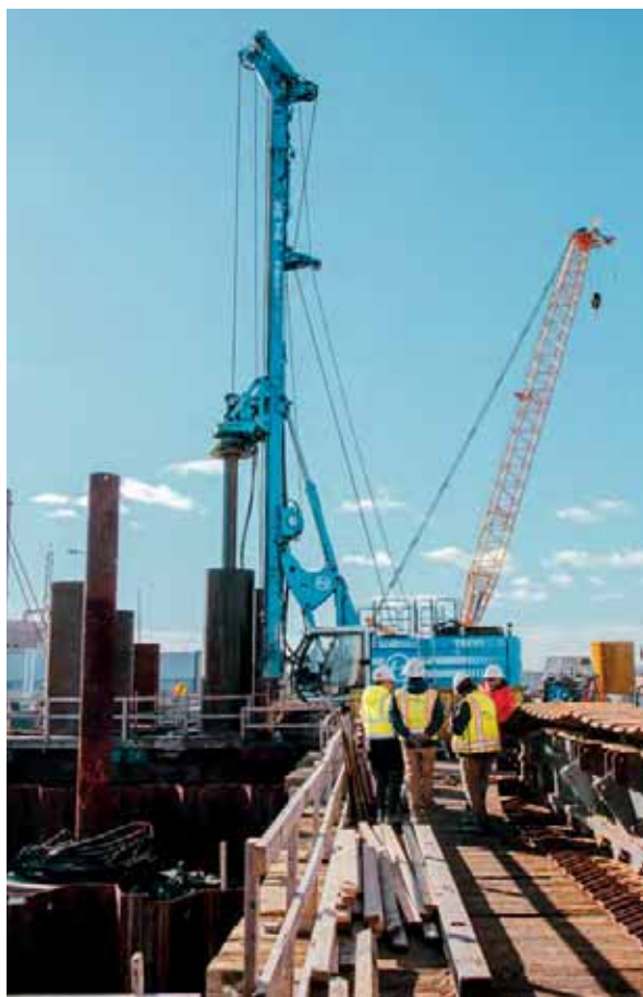
Belden Bly bridge project | MA, USA
